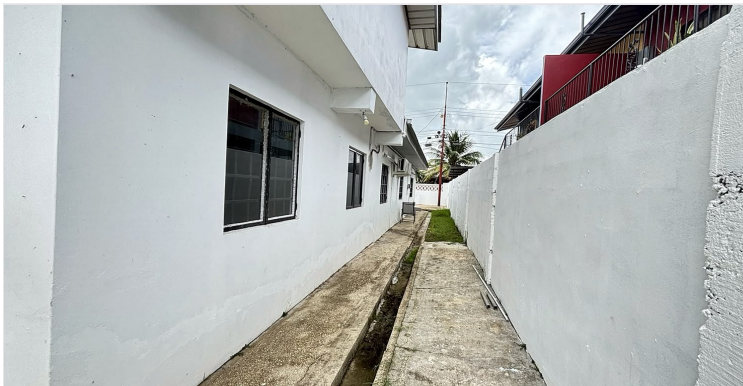
Apartment Side Access
